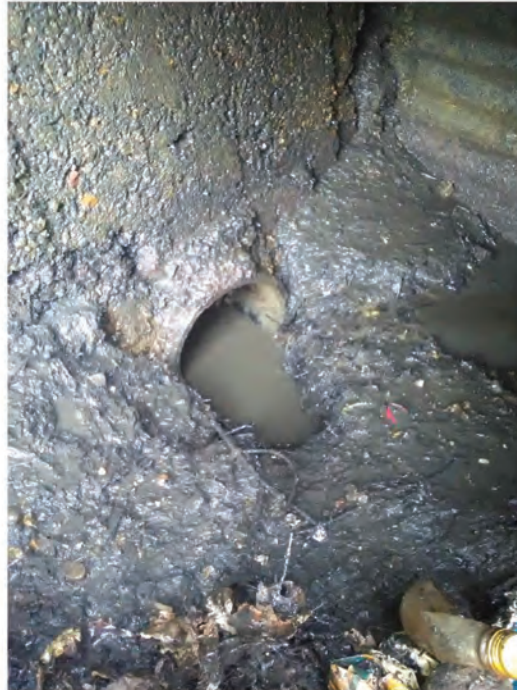
Image A:- View of the exposed outfall pipe from ditch
