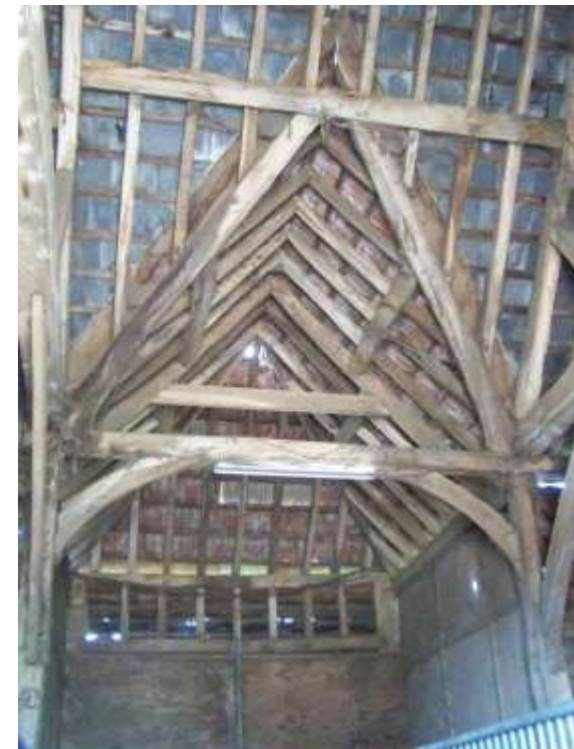
Figure 9: Interior, Looking South
