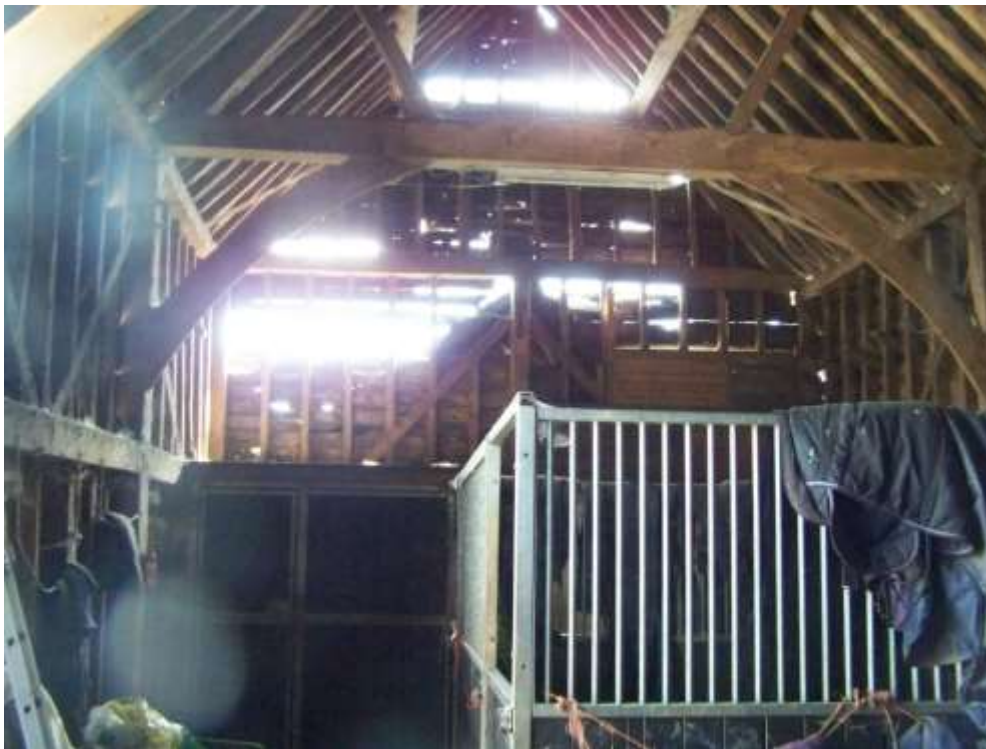
Figure 8: Interior, Looking East
