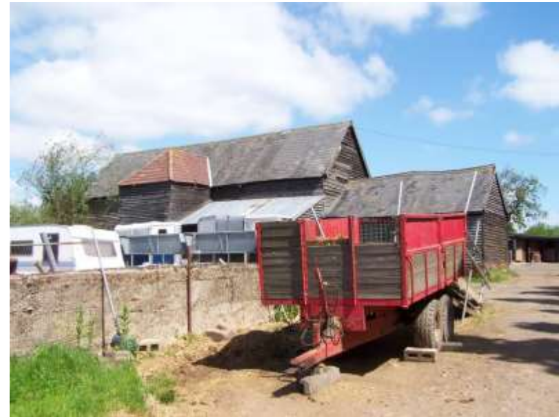
Figure 5: The Barn, from the southeast
