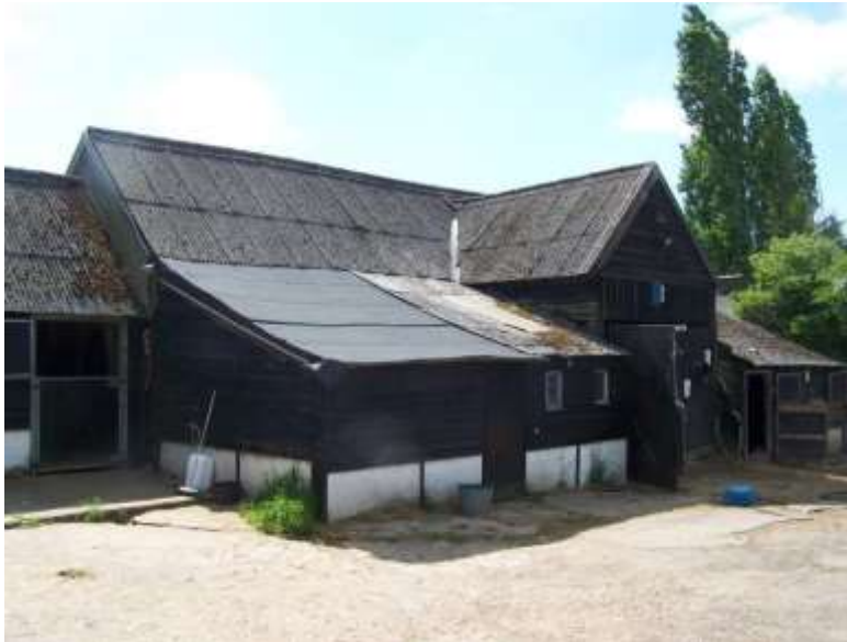
Figure 6: Barn to East of the Listed Building, Exterior
