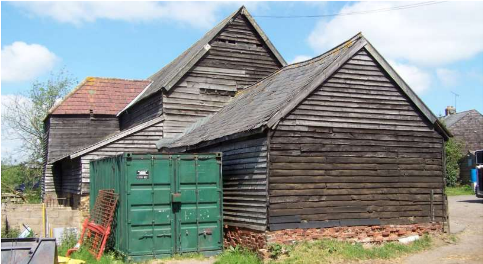
Figure 2: The Grade II Listed Barn, from the east
