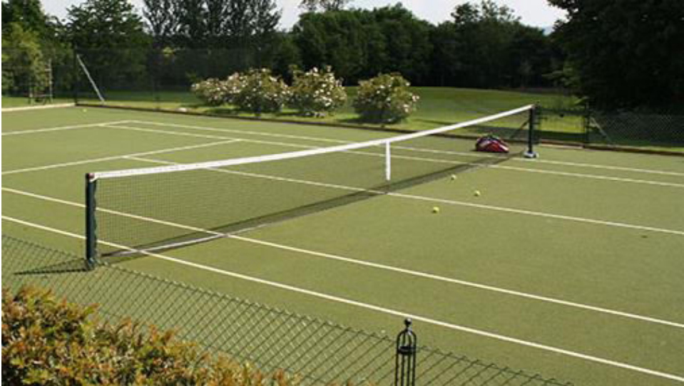
The sand filled synthetic grass court surface blends well with adjacent lawn.
