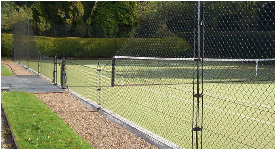
2.75 metre high fencing at both ends but dropping down to the lower height of 0.9 metres along the sides.
