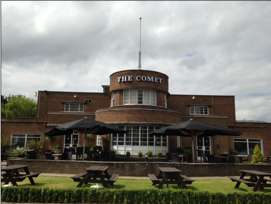
Plate 10. Front view of Comet Hotel facing south-west.
