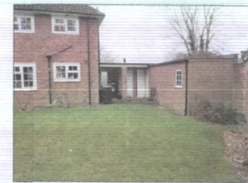
Photographic Image Property as viewed from rear garden
