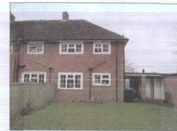
Photographic Image Property as viewed from rear garden
