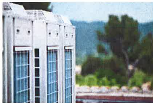
ASHP Outdoor Units
