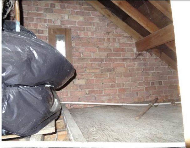
Photograph 16: Access point within the building loft space.
