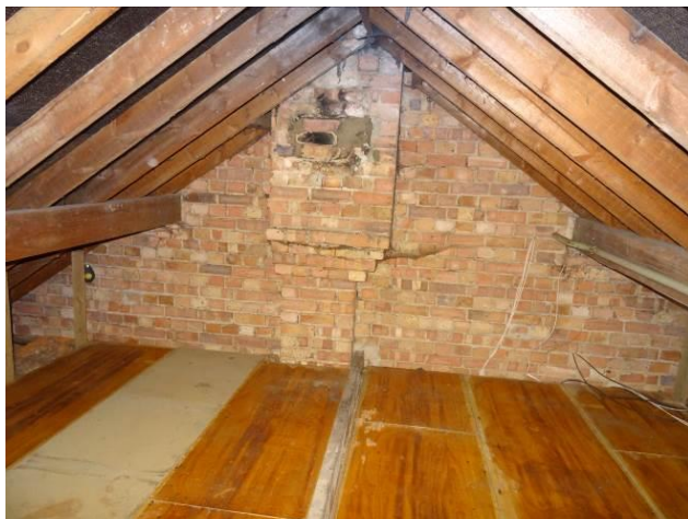
Photograph 17: Loft space of the building
