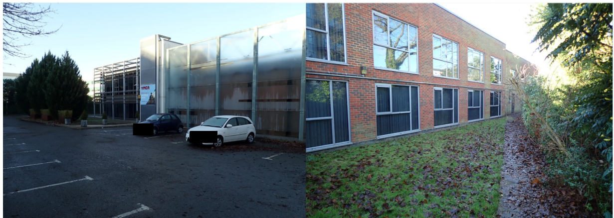
Photograph 1 (left): Front (south-east) elevation of the former hotel looking west; Photograph 2 (right) – Side (northeast) elevation looking north-west.
