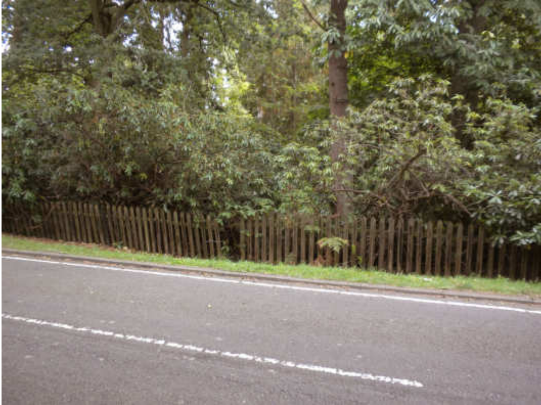
Existing front boundary fence and tree screen to The Warren
