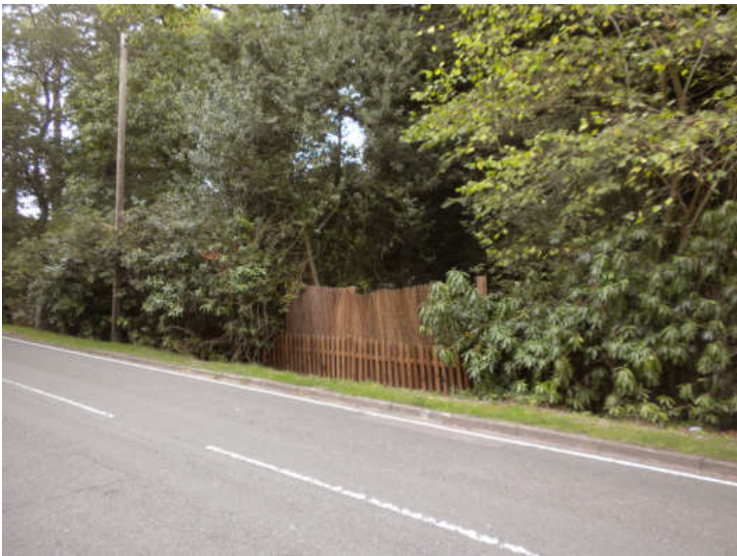
Recently repaired front boundary fence to The Warren
