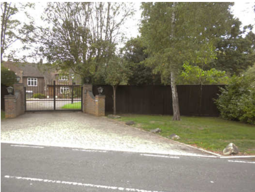
Brick entrance piers, metal gates and 2.0m high close-boarded fence to 1 Carbone Hill
