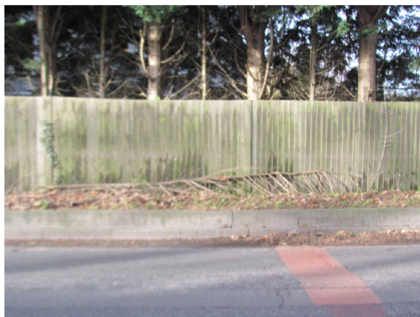
PHOTO OF EXISTING FENCE FROM COOPERS LANE
