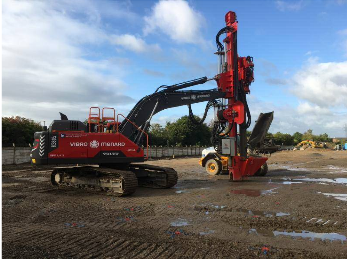
Figure 3 – Example of VSC installation on site
