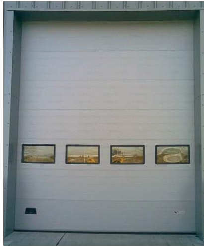
Image 8; Typical vehicular access door - aluminium colour RAL 7016 – anthracite grey
