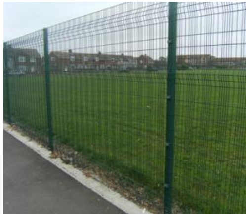
Image 15; Typical paladin boundary security fencing polyester powder coated steel – colour RAL 6005 – green
