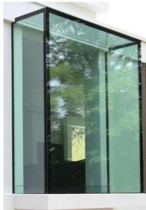
Image 11; proprietary orial feature windows to first floor office – frameless clear self finished
