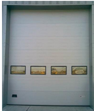
Image 14; Typical vehicular access door - aluminium colour RAL 7016 – anthracite grey
