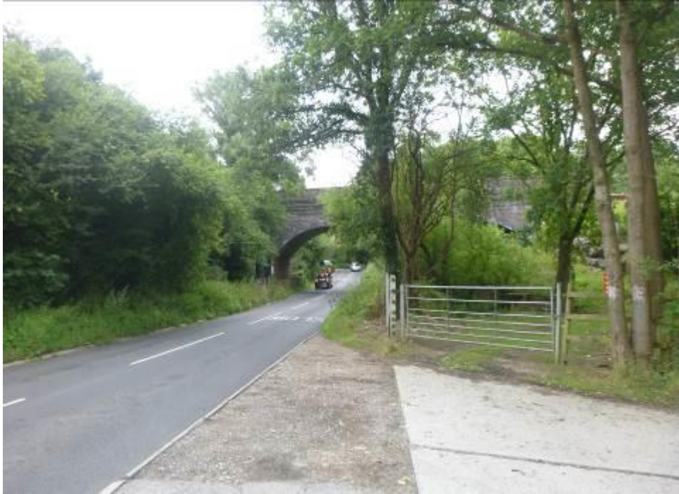
Photograph 10 Showing Newgate Street Village road and the railway line
