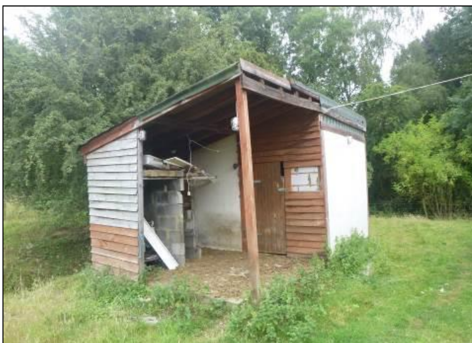
Photograph 7 Showing the outbuilding on the eastern section of the site
