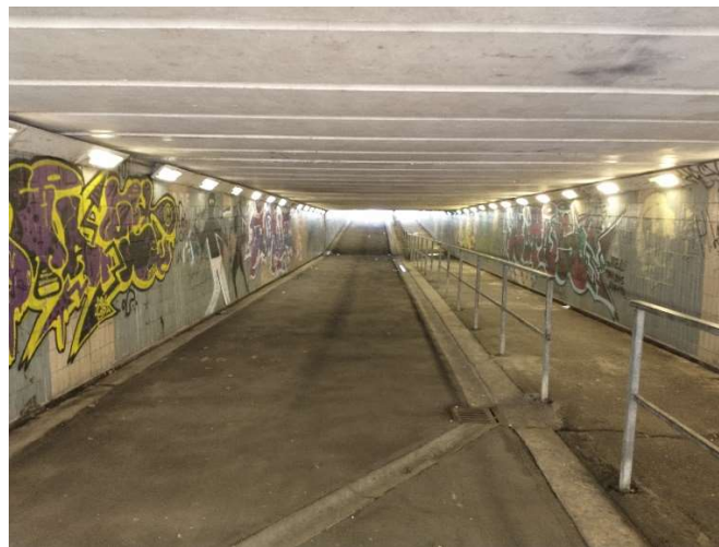
Figure 4 Subway under Comet Way
