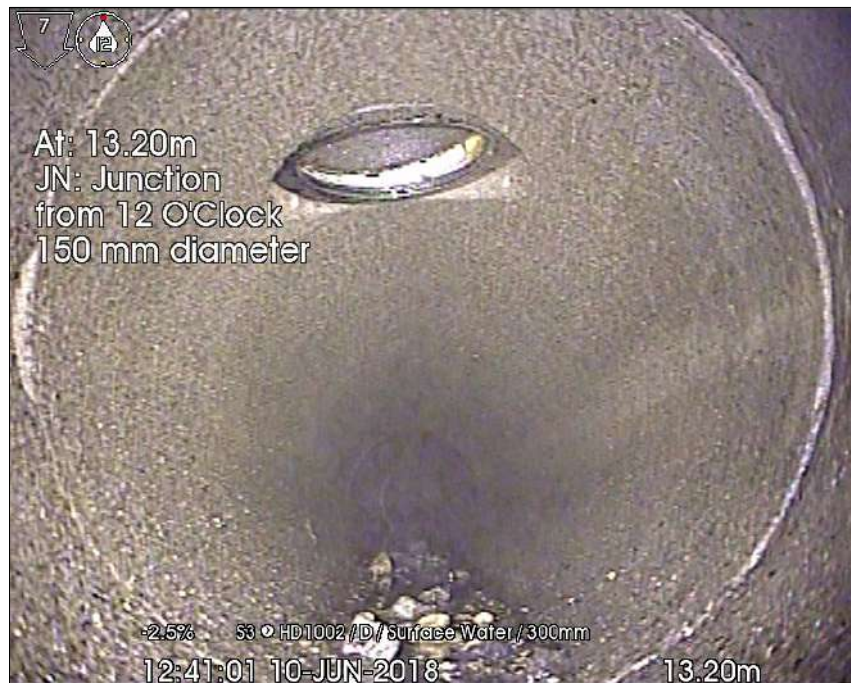
Photo: 1 - S3 downstream to HD1002_13-20m_124101.jpg 13.2m, JN: Junction from 12 O'Clock 150 mm diameter
