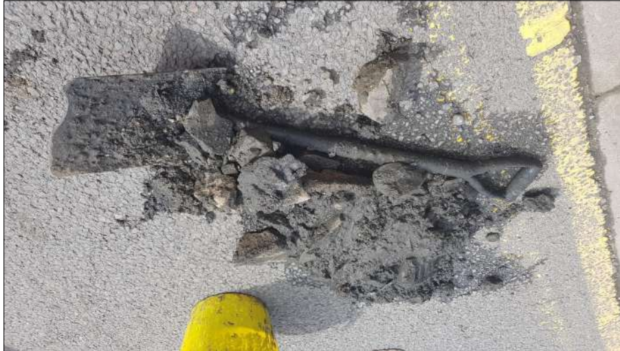
Photo: Hatfield 4.jpg 0m, General condition photograph
