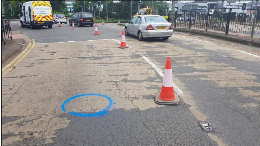
Photo: Hatfield 3.jpg 25.32m, General condition photograph
