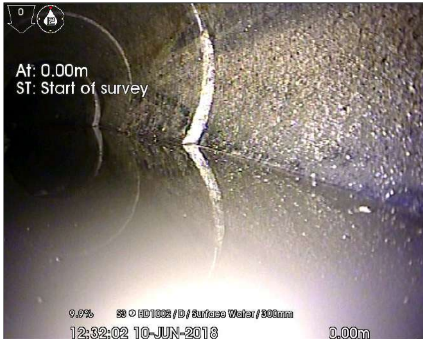
Photo: 1 - S3 downstream to HD1002_0-00m_123202.jpg 0m, ST: Start of survey
