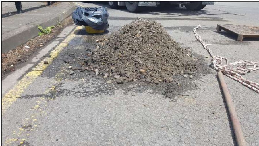
Photo: Hatfield 2.jpg 0m, General condition photograph
