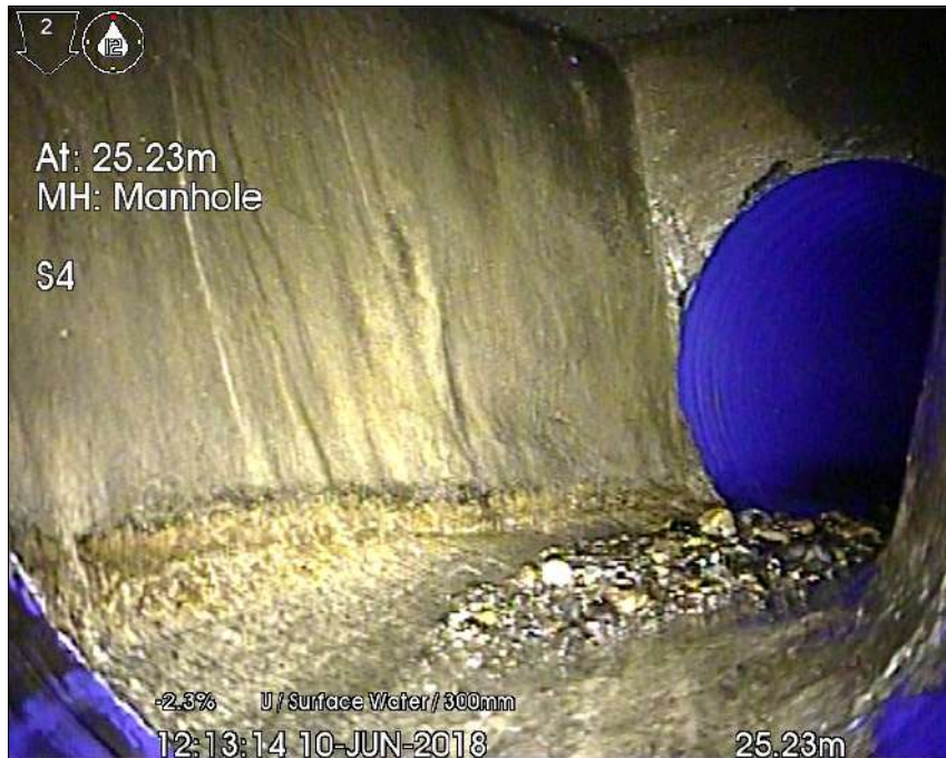
Photo: 2 - S3 upstream to S4_25-23m_121314.jpg 25.23m, MH: Manhole S4
