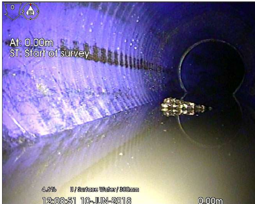
Photo: 2 - S3 upstream to S4_0-00m_120851.jpg 0m, ST: Start of survey
