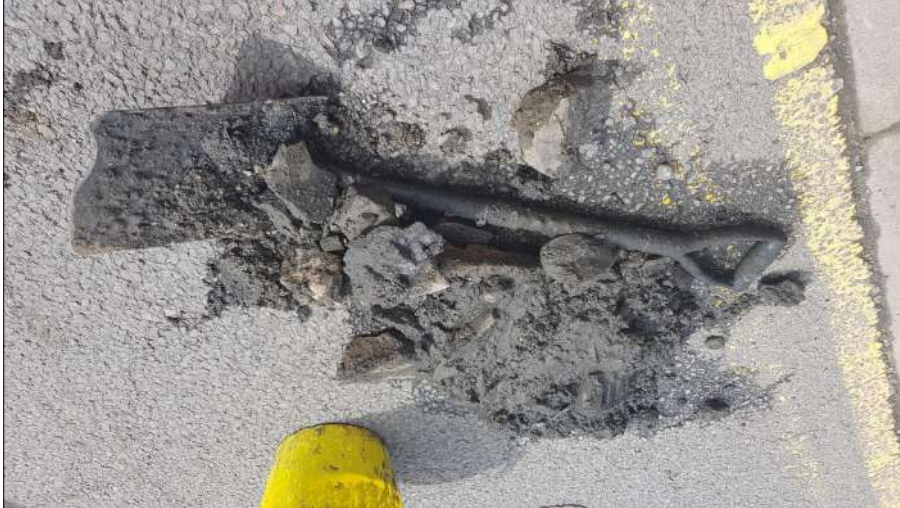
Photo: Hatfield 4.jpg 0m, General condition photograph
