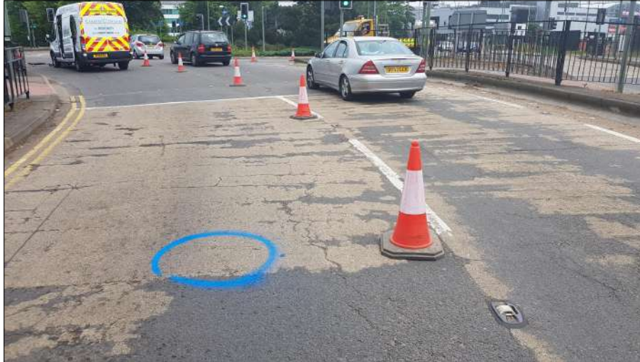
Photo: Hatfield 3.jpg 25.32m, General condition photograph
