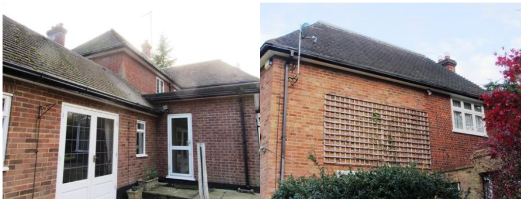
Photographs 1 – 4: Front, rear and side elevations
