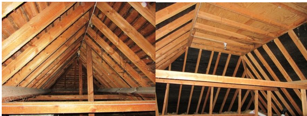
Photographs 5 – 6: Internal roof void
