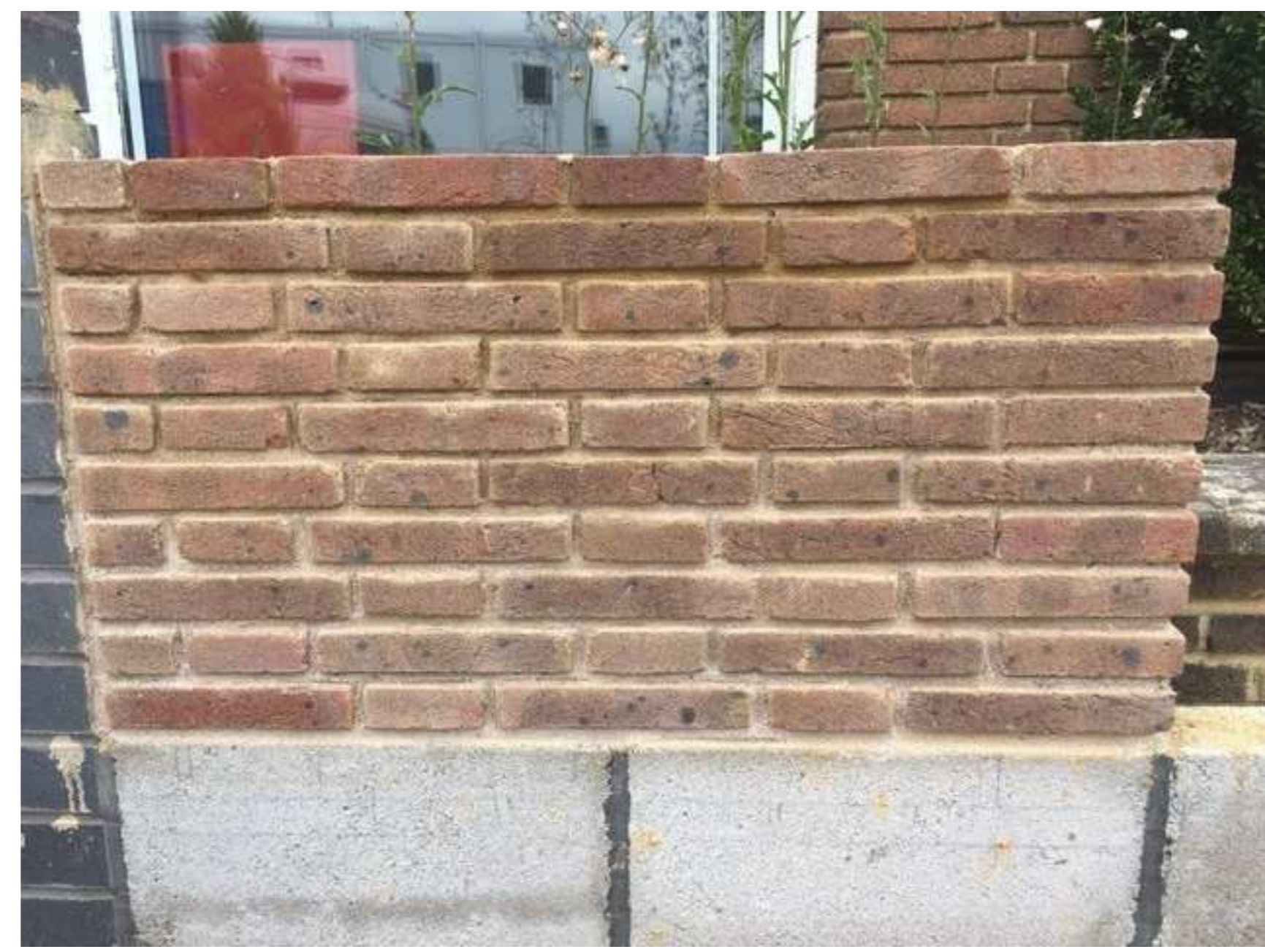
Proposed Heritage brickwork sample panel to match existing Heritage brickwork, bond and mortar colour. Brickwork reference H.G Matthews 'Brown grey bottom of kiln'
