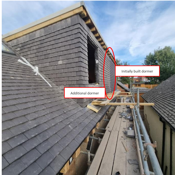
Additional dormer walls
