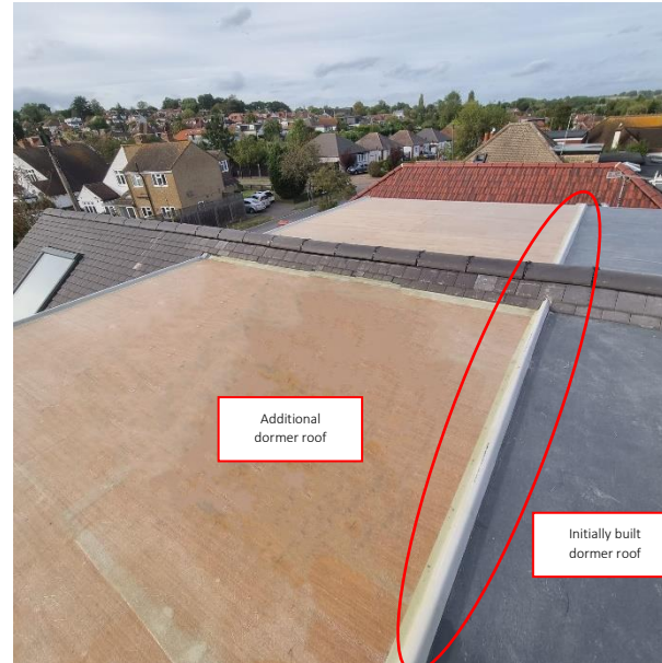
Additional dormer roof
