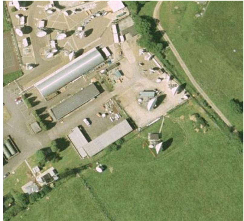
Plate 11: 2000 aerial photograph of the area of proposed development and its immediate surrounds demonstrating the presence of transmission equipment within the area (Source: Google Earth).
