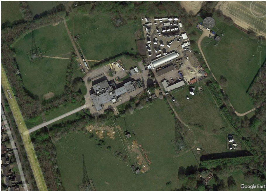
Figure 2.1 Aerial View of Brookmand Teleport Site
