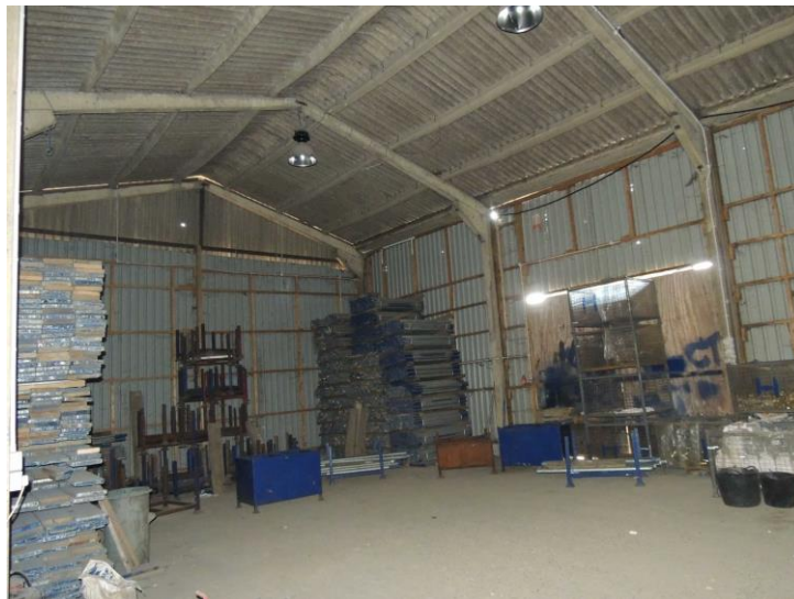
Photo 7: Interior of Building 3
