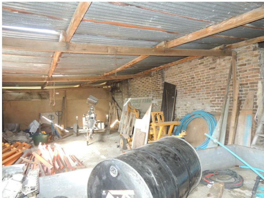
Photo 14: Area beneath the lean-to
