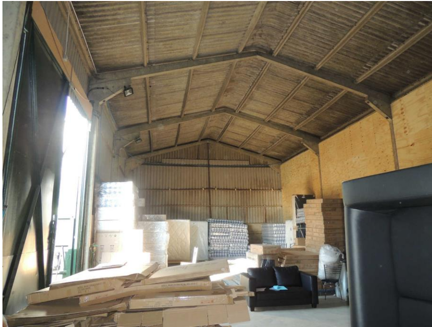
Photo 4: Looking south-westwards in Building 2
