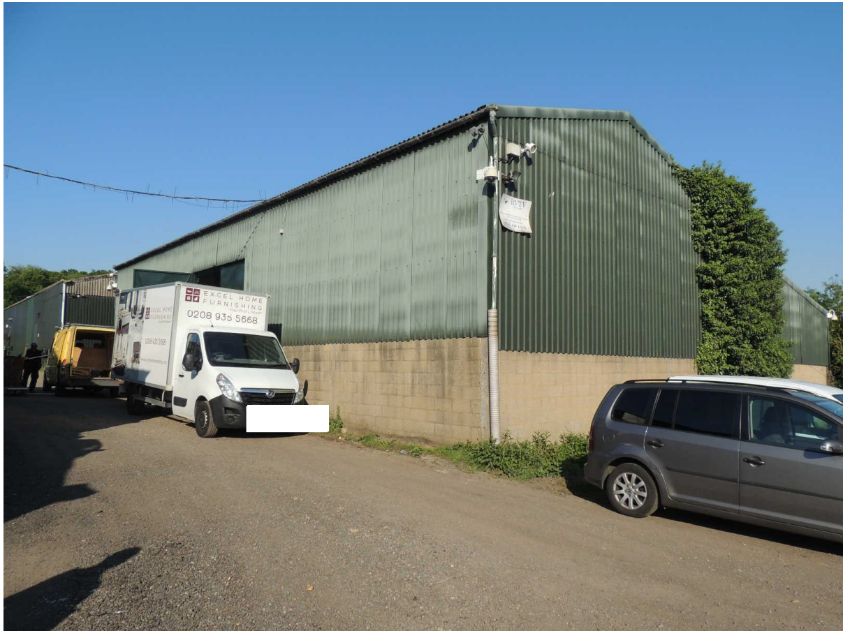
Photo 1: Building 2. The buildings at the site comprised warehouses and open barns used for storage
