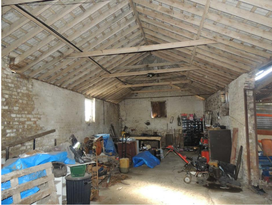
Photo 15: Looking north-eastwards along the single-storey brick barn
