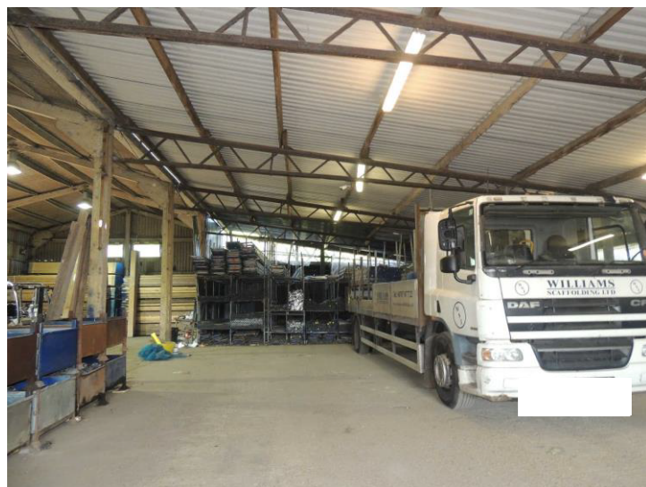
Photo 8: The lean-to area had a metal sheet roof
