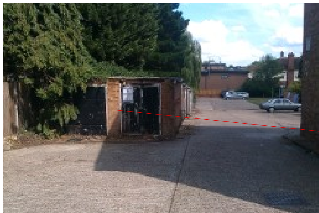
view of site, slackspace, access and shed (west facing)
