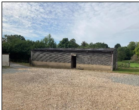
Photograph 5: View of Building D and associated hardstanding.
