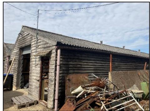
Photograph 4: View of building E with confirmed roost.
