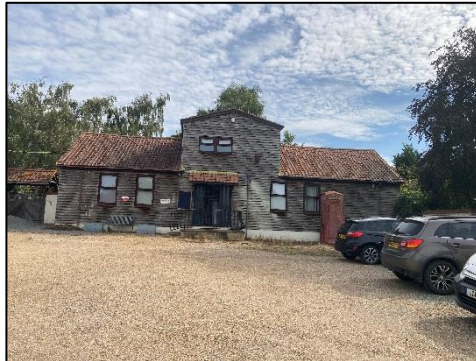
Photograph 1: View of Building B, with confirmed roost.
