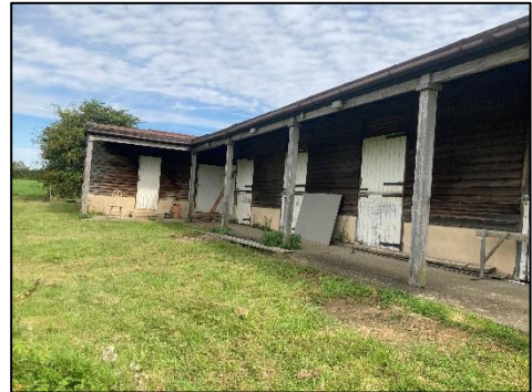
Photograph 2: View of Building F, former stable block with confirmed roost.
