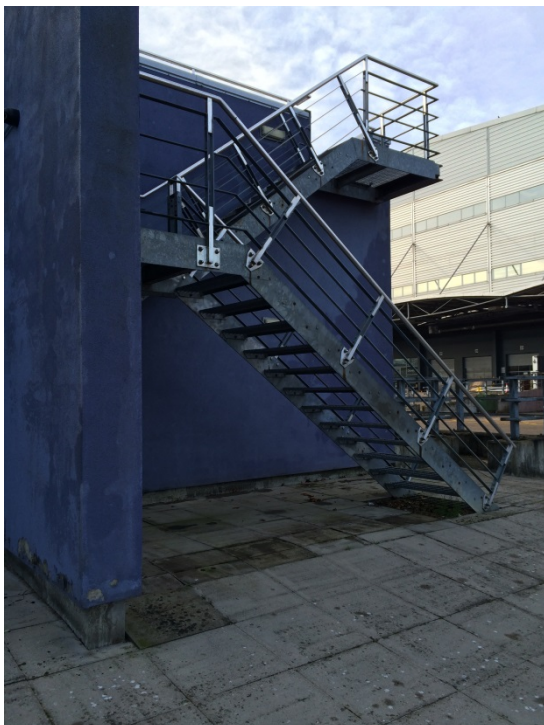
North End 1 st Floor Fire Escape Stairs
