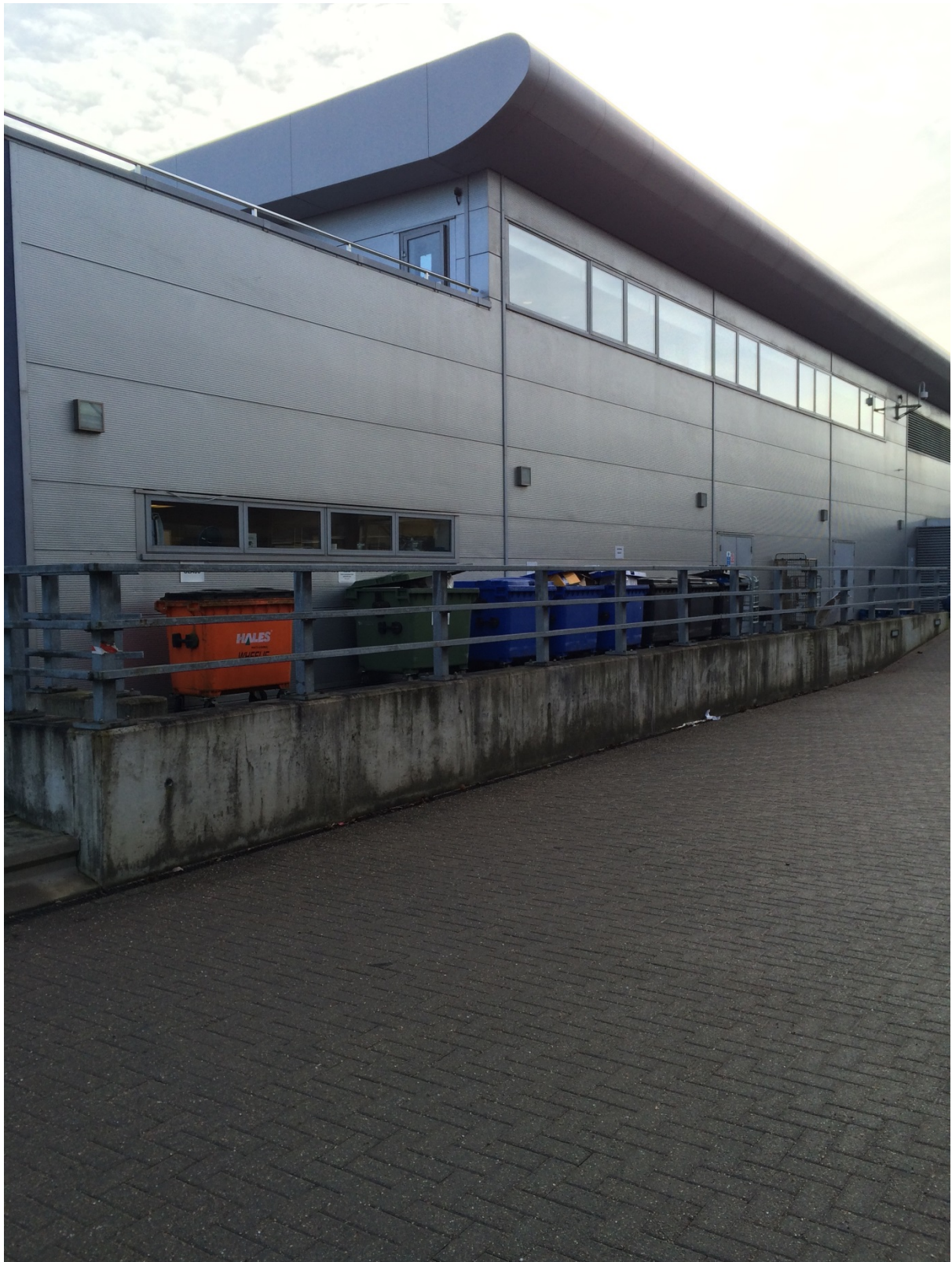
North End Rear Location for First Floor Raised Toilet Block
