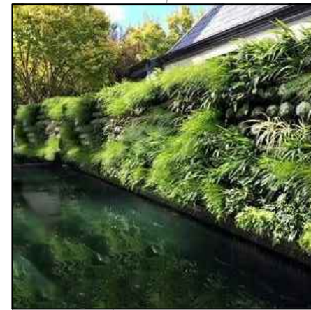
SOUTH FACING HYDROPONIC MODULAR LIVING WALL PLANTER UNITS FITTED TO SYSTEM SUPPORTING FRAME AUTOMATED PROGRAMMER PUMP FLOW RATE AND DOSE SET POWERED BY pv/BATTERY STORE
