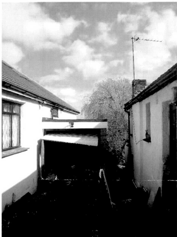
01 FRONT OF GARAGE - FACING NORTHAW ROAD
