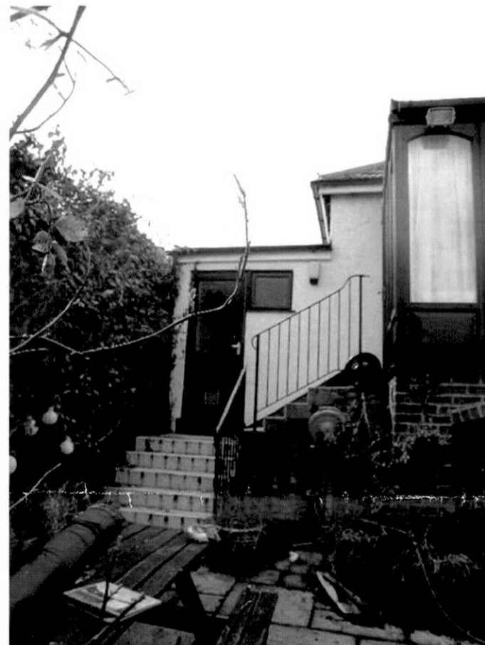
02 REAR OF GARAGE - DOOR & WINDOW TO GARDEN STORE
