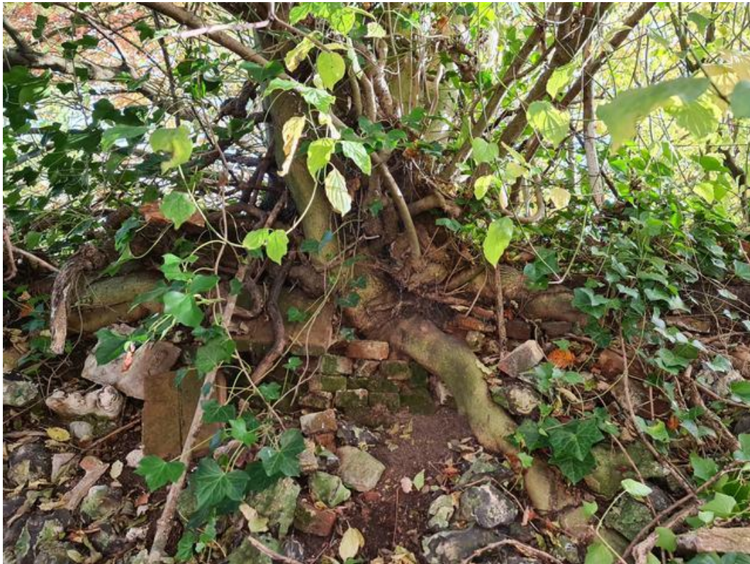
Image 7 T308 the multi stemmed ash tree growing on top of the existing wall.
