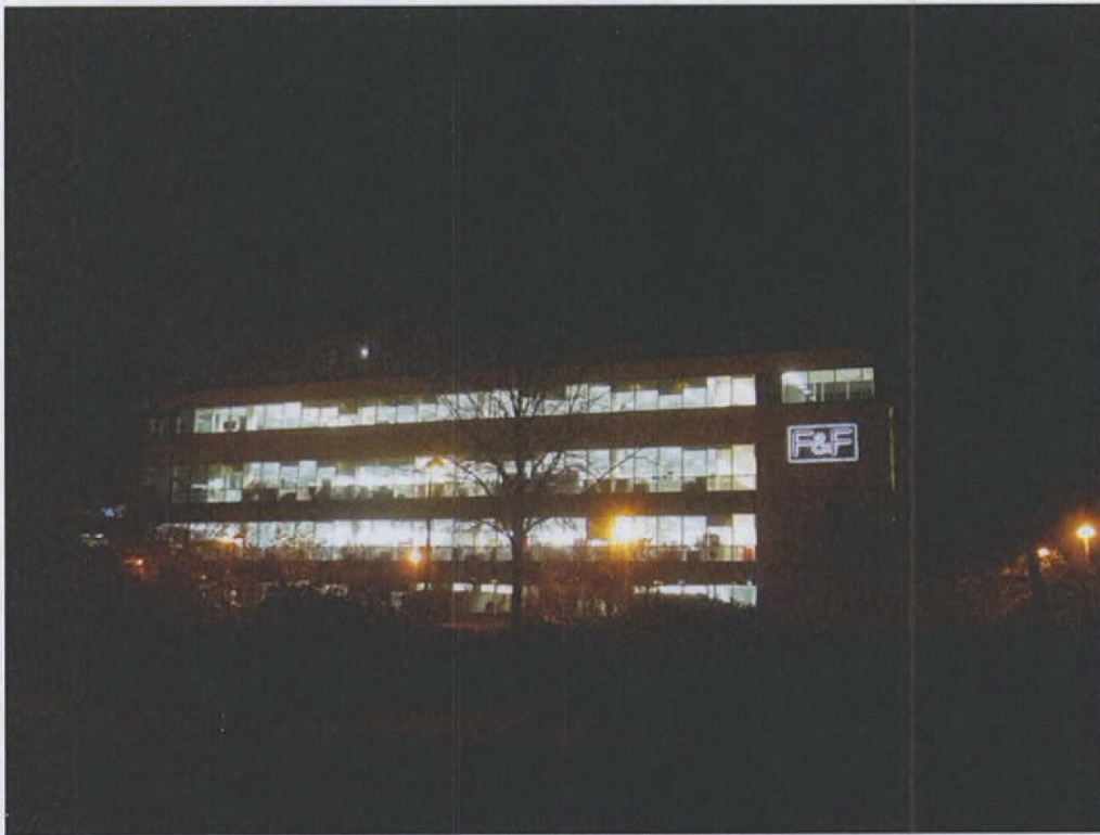
Photo 7: View from Mosquito Way of F&F Building with illuminated sign
