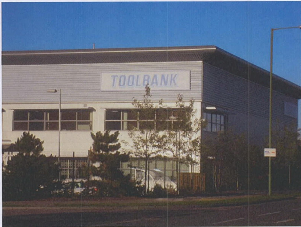
Photo 6: Toolbank Building, with fascia sign
