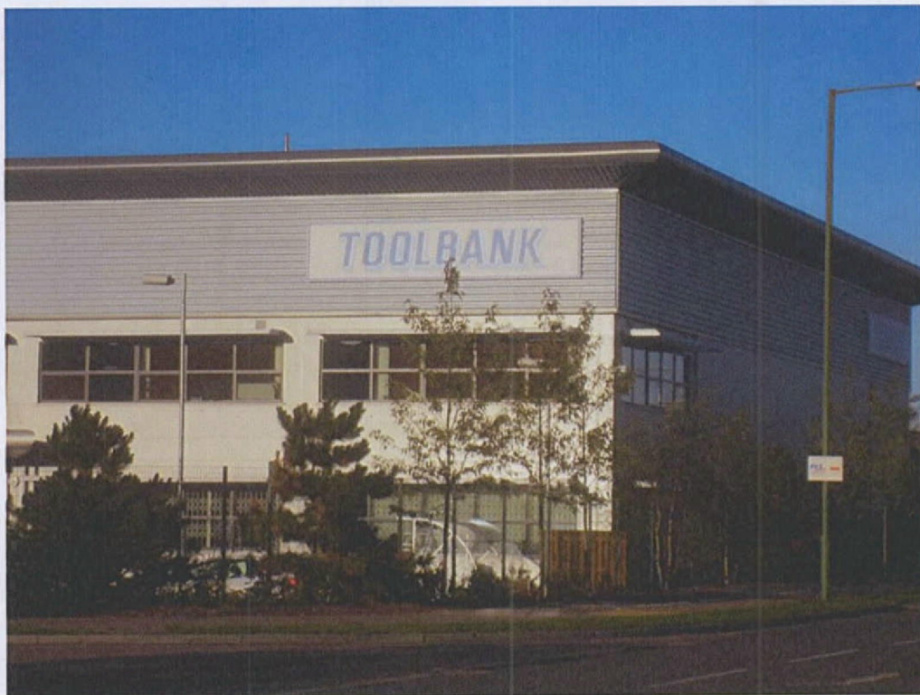
Photo 6: Toolbank Building, with fascia sign
