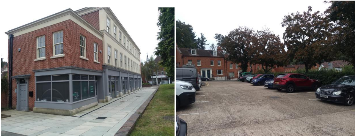
Figures 1 and 2: Images of the hardstanding forming a car park and walkways
