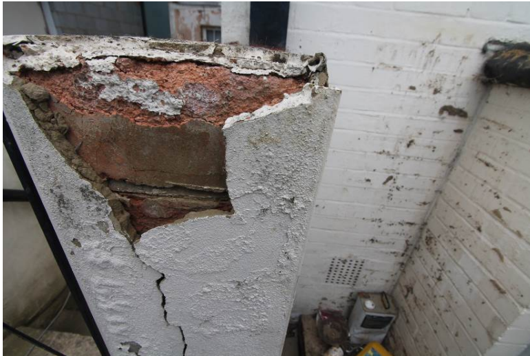
8.0 – (7762) – Point for sample 2 on dwg 6842-77-P0. area with lime render
