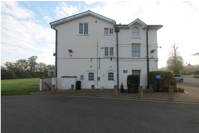
Left side (west) elevation of Oshwal House
