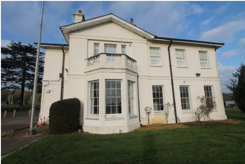
Right side (east) elevation of Oshwal House
