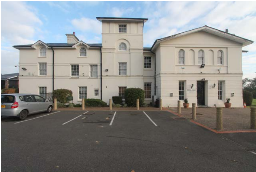
front elevation (south) of Oshwal House
