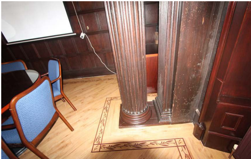
2.2 – (4036) – Board Room Figure 1.0 Room 2 detail of the right-hand side column
