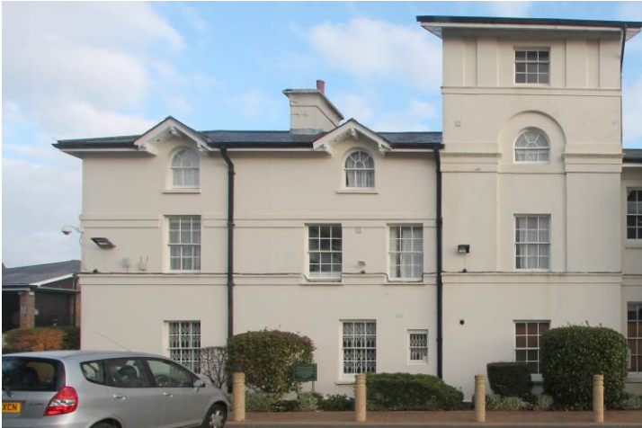
southwest wing and tower: front elevation (south) of Oshwal House
