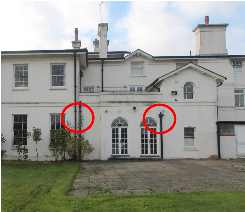
Details of the existing cast – iron pipes
