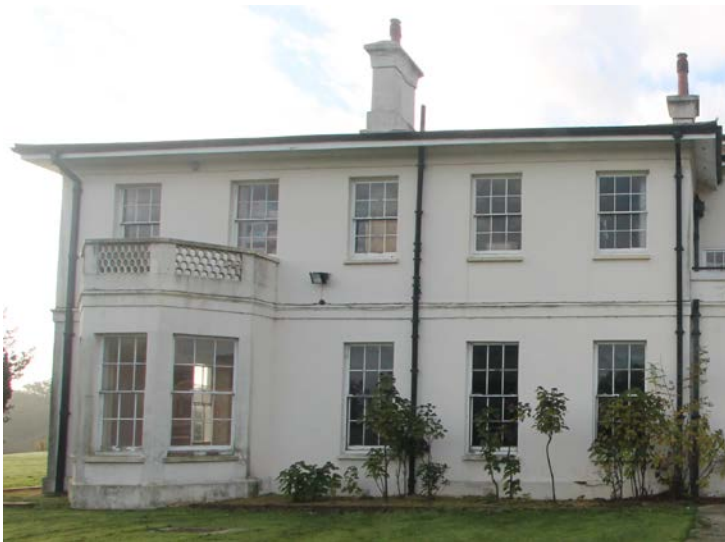
original house: rear elevation (north) of Oshwal House
