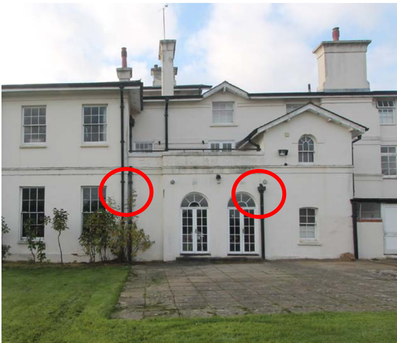
Details of the existing cast – iron pipes
