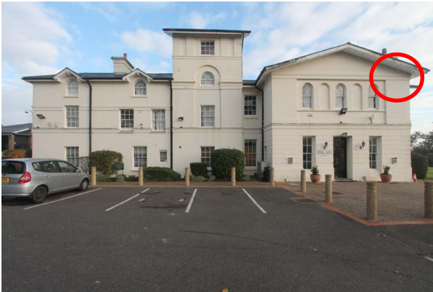
Detail cornice on the front elevation which has been used on the eaves of the extension (see drawing 6842-40-P0)
