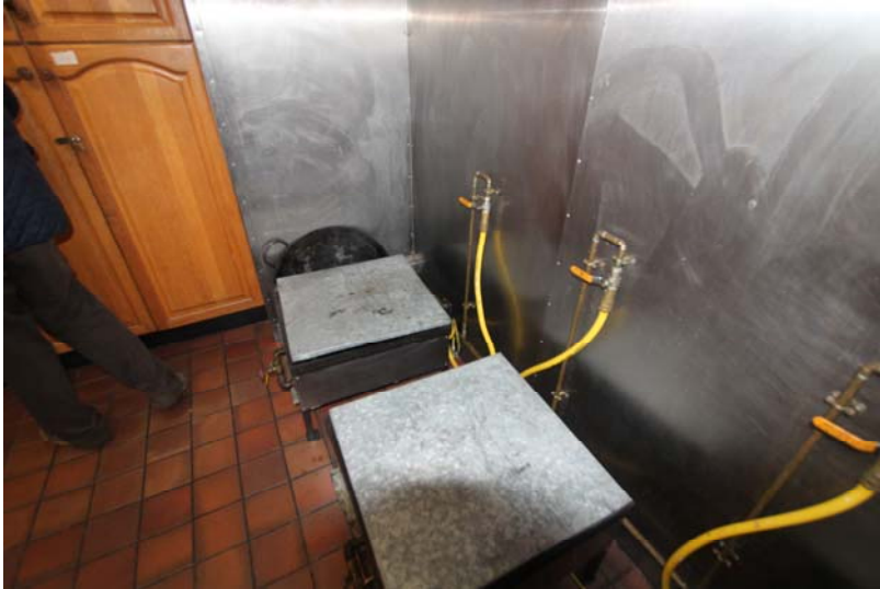
Detail of the existing kitchen
