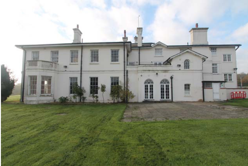
Rear (north) elevation of Oshwal House
