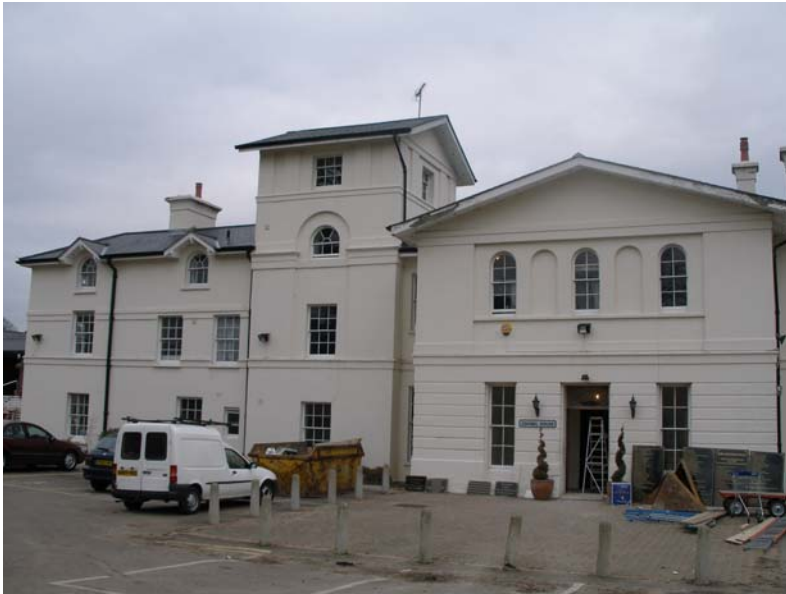
front elevation (south) of The Hook House
