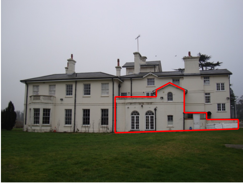
Rear elevation of The Hook House and the old rear extension to the original House
