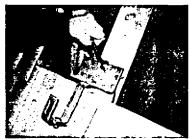
After removing the tiles where necessary, assemble the hooks to the frame with the relevant screws. Respect a distance of 1,20 m maximum between two hooks.
