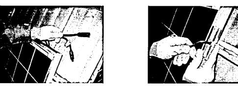
Clamp the module to the profile. Don't forget to interconnect the modules strings step by step
