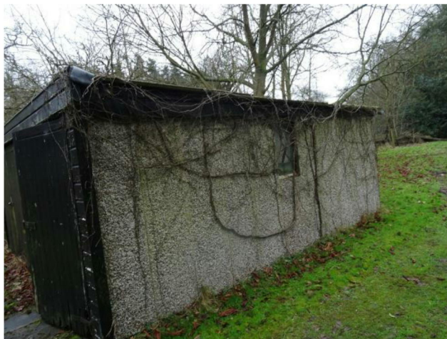
Photograph 5 Building 4 in the south of the site.
