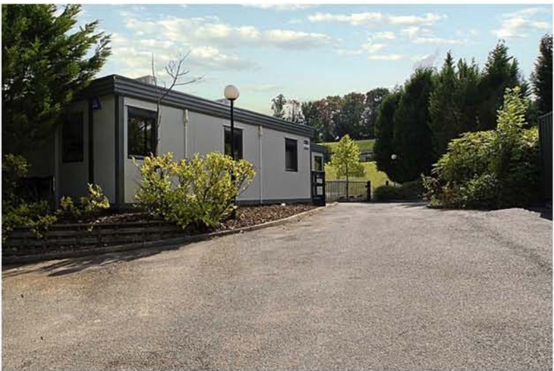
fig. 6 - example of external cladding
