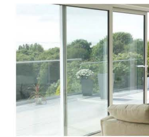
WHITE ALUMINUM PATIO DOORS TO REAR
