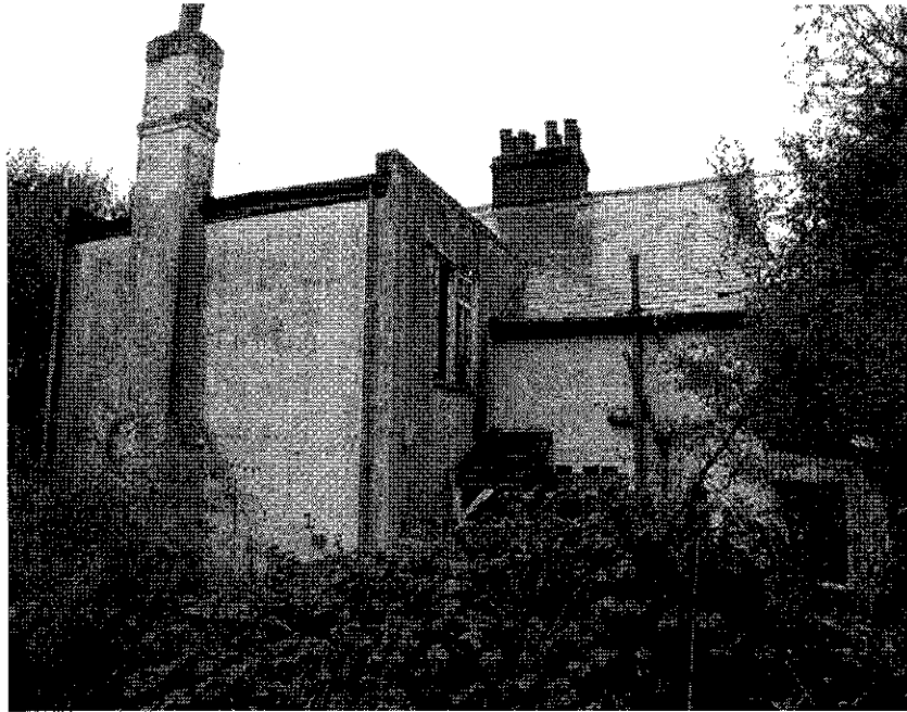
Plate2: The only side of the cottages which is fully viewable.
