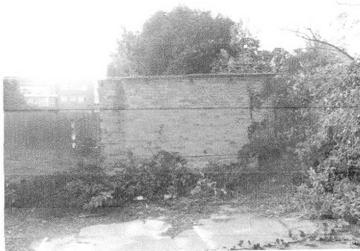
Site North Eastern Corner
