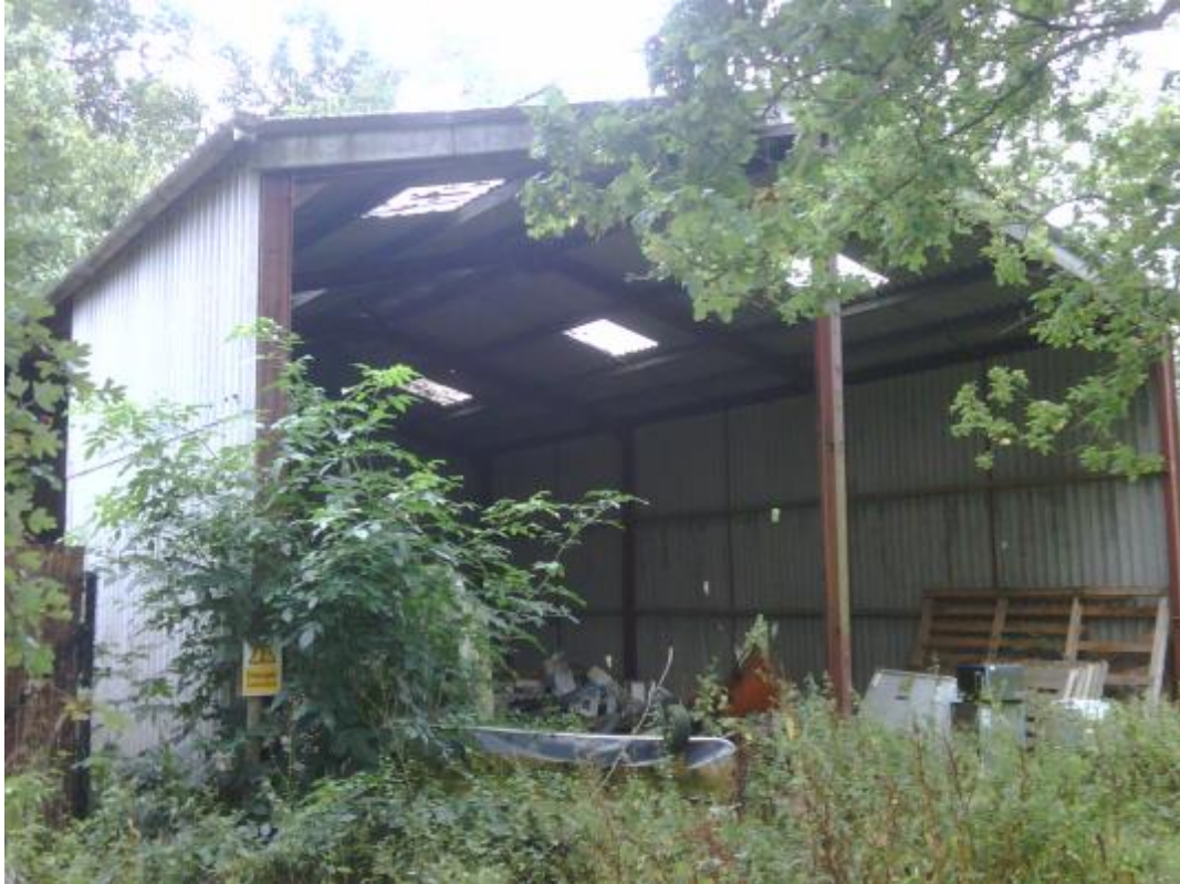
Existing store building
