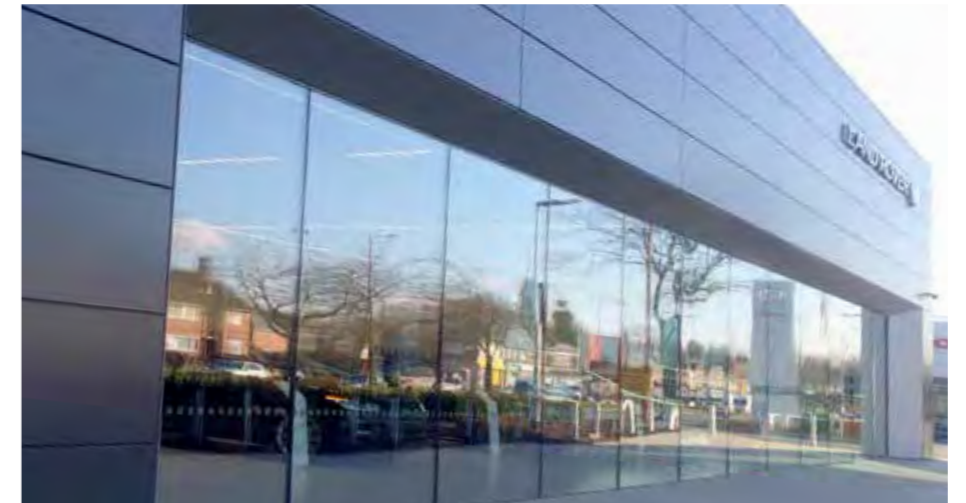
'Sunshine Grey' cladding with structural glazing to showroom
