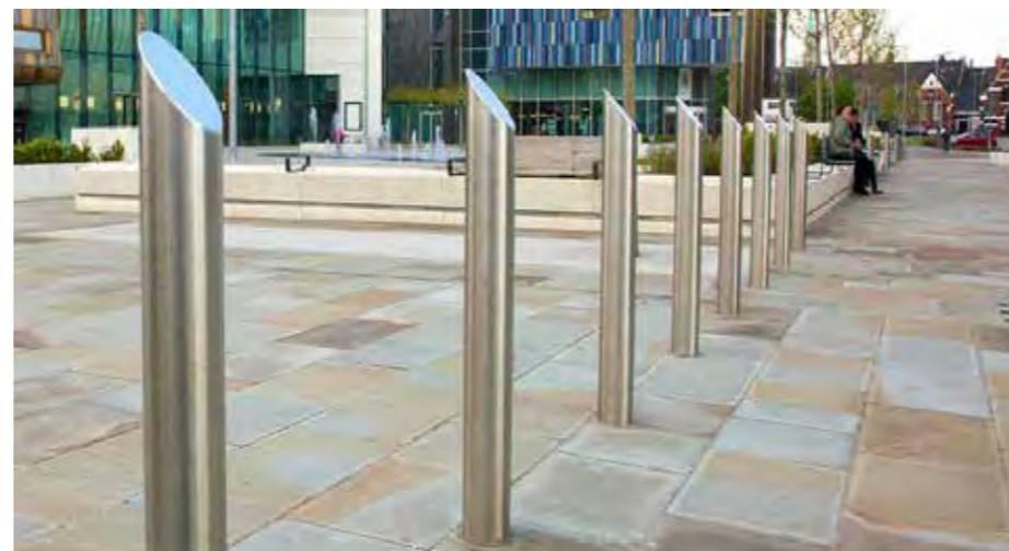
Stainless steel security bollards around customer facing perimeter
