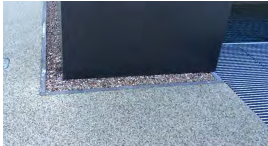
Resin bonded gravel path with gravel margin and external wipe off matting
