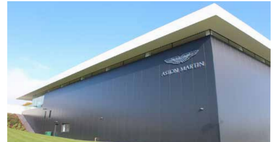
South, main road and entrance facade to be white render, black cladding on all other elevations
