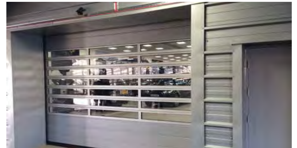
Light grey horizontal trapezoidal cladding and workshop doors
