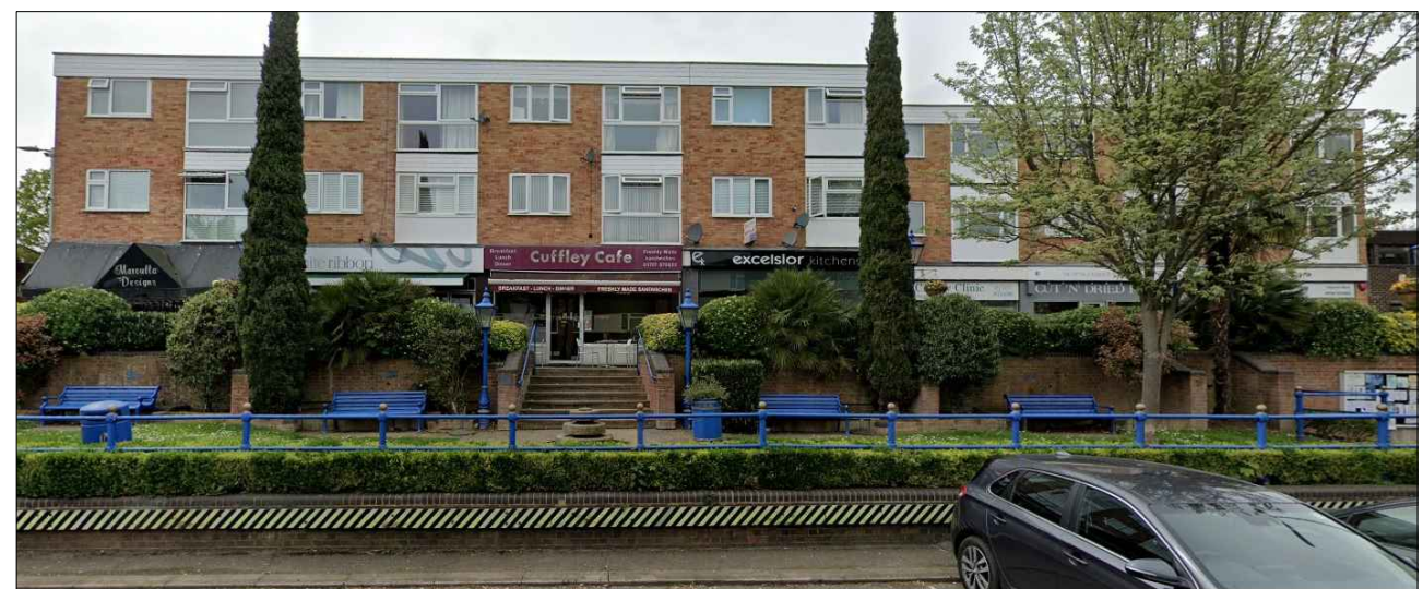
PRE-EXISTING FRONT ELEVATION - APRIL 2018
